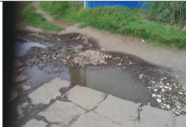
Figure 18: Leaking sewer pipe, Madwaleni Hospital (EC), 2016
