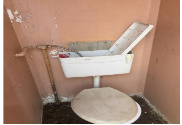
Figure 10: Public toilets, Mothotlung Police Station, 2016
