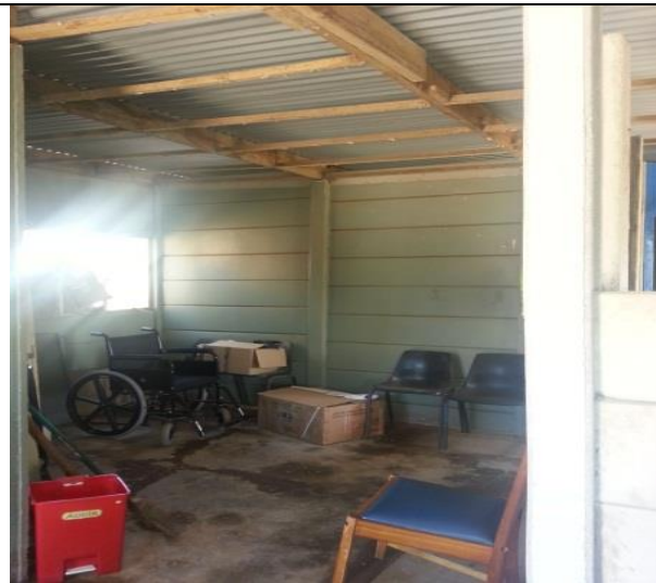
Figure 5: Outside area used for storage at Isolomzi Clinic, 2014
