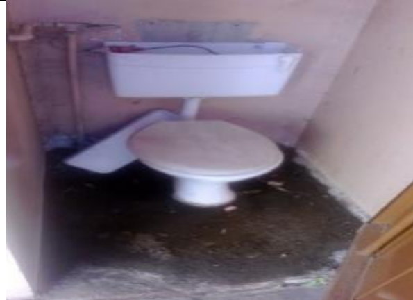
Figure 9: Public toilets, Mothotlung Police Station, 2015
